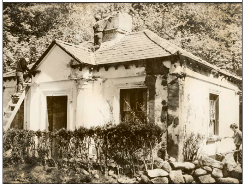
The Gate Lodge under repair in 1970's
